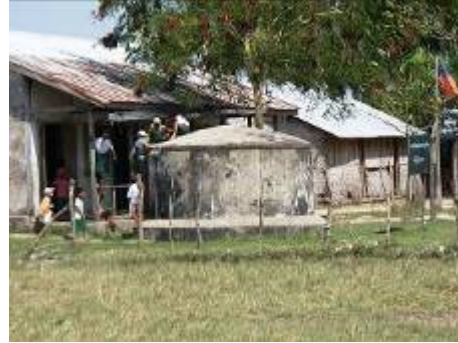
Rain Water Collector Tank – School in Laputta Township
